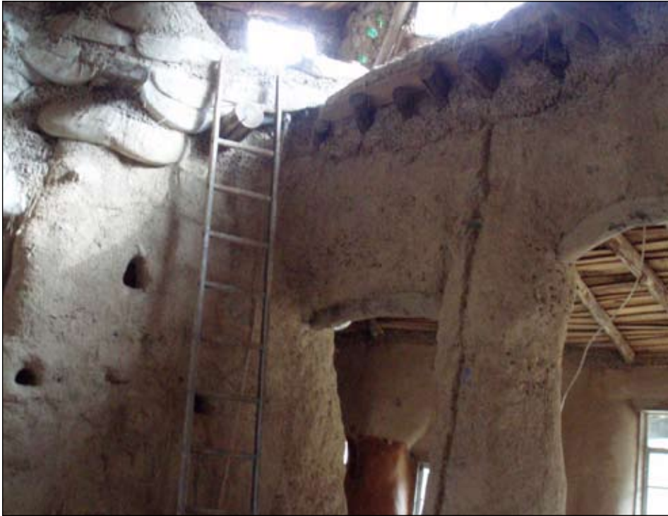
Reaching new heights. A ladder in a strawbale building at The Farm's Ecovillage. Photo by Jessica Farquhar
